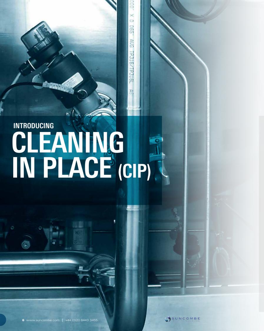
CIP or in its full form, Cleaning In Place, is defined as techniques to clean process equipment without dismantling and with minimal operator involvement.
